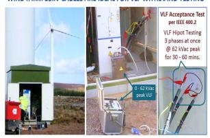
Cable system is new. Needs VLF AC Withstand test to find workmanship errors on splices and terminations and possible cable installation damage. VLF it!
